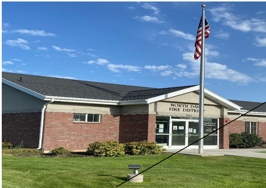
West Point Station 41 NDFD Headquarters
