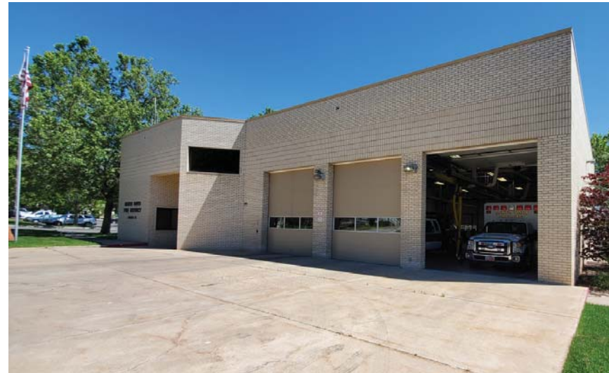
FRONT (NORTH) VIEW
